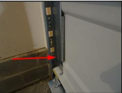
The bracket on the second panel is bent outward. This will likely effect the door function in the future. All systems listed should be evaluated and repaired as needed by a general contractor to ensure that all systems are functioning as intended.
