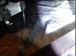
The insulation is compressed or displaced. The effectiveness of the insulation is reduced when displaced or compressed. Improper insulation installation could result in condensation, over heating of the building components, and inadequate conditioning of the living areas. A licensed general contractor should be consulted for repair/replacement.
