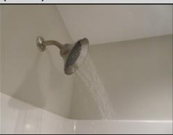
The water pressure is low at this fixture. This can be from something as simple as a clogged aerator or shower head. It could also be a faulty faucet or a larger plumbing issue. A licensed plumber or general contractor should be consulted for the repair.
