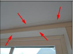
A stain was found here on the trim around the window which measured as dry with a moisture meter. This could reoccur at anytime. A licensed general contractor should be consulted for the evaluation and repair.
