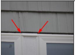
Typically, the mullen for the windows by the master bedroom has a J-channel that runs across both windows in one piece to avoid leaks. The areas by the arrows may allow water down the mullen and cause decay. Builder evaluation is needed.
