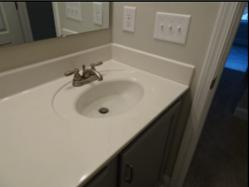
The sink drain was noted to drain slow when filled above halfway. This could be a clogged trap or a more significant plumbing issue. A licensed plumber should be consulted for repair.
