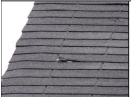
The shingles have been damaged from foot traffic/ladders/tools and are in need of replacement like this on the front left. The number of damaged shingles were too many to give specific locations. Damage to the ballast (small rocks) removes the layer that protects the water proof layer underneath. This will result in premature failure of the damaged shingles. A licensed roofing contractor should be consulted for a full roof evaluation of the entire roof covering system.
