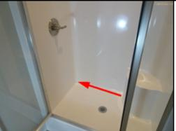
The fiberglass/acrylic tub has a break in the surface that exposes the structural matt. The chip could allow water to penetrate under the surface and possibility result in leaks. A licensed general contractor should be consulted to determine if the tub surface can be repaired or if replacement is needed.
