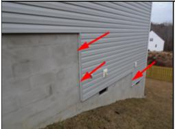
The siding is not covering the wall structure. This should be repaired or replaced by a general contractor to prevent damage from water entry into the wall. Future hidden damage is possible.
