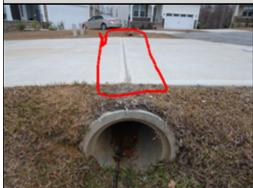
The driveway is thinner than the typical 4 inches and is much more likely to crack in this area. The round culvert does not offer even support for the slab. A licensed general contractor should be consulted for further evaluation, to determine the extent of the damage, and to make necessary repairs.
