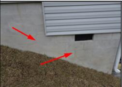
Closed/Open cracks were noted in the foundation of the home. Cracks in the foundation indicate a deficiency in the foundation, footing, or supporting soil that can change and worsen if it progresses over the life of the home. An engineer should be consulted to determine the significance/cause of the cracks and outline any necessary repairs.
