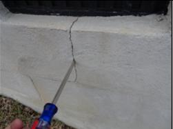
Additional Photograph: This is a photograph of the crack closest to the back right corner. This is larger than what is common for a new home. The steep hill makes the crack more of a concern needing evaluation. An engineer should be consulted for a complete evaluation, to determine the significance of the concern and outline necessary repairs.
