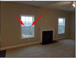
The window needs repair to ensure proper operation. The window did not properly latch. All windows should be evaluated as repairs are made. A licensed general contractor should be consulted to review the installation and repair as needed to ensure safe and secure operation.
