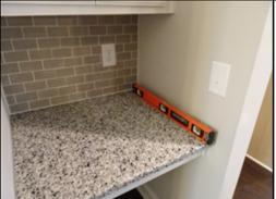
This counter is significantly slanted downward. All systems listed should be evaluated and repaired as needed by a general contractor to ensure that all systems are functioning as intended. The contractor should consult specialist in each trade as needed.
