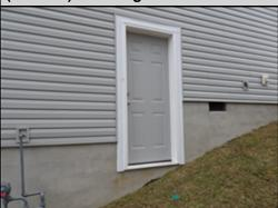
Having no step near the crawl space door is a fall hazard. A licensed general contractor with experience in landscaping and grading should be consulted to evaluate and correct the grading as needed.
