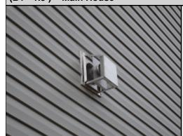
The trim is not properly installed by the exhaust. There is no flashing/J-channel and no flat trim panel which diverts water away from the home and down the siding. The caulk used here is not designed to be installed this thick and is not designed to hold the vinyl siding (when applicable) in place. This should be repaired or replaced by a general contractor to prevent damage from water entry into the wall. Hidden damage is possible.
