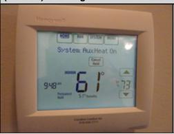
The heat pump was not operating properly at the time of the inspection. The auxiliary heat designed to assist the unit in extreme temperatures did not function in auxiliary or emergency mode. A HVAC contractor should be consulted for a complete evaluation and to make necessary repairs to ensure safe, reliable, and proper operation of the HVAC system.
