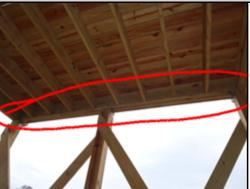
The joist have only been nailed from the exterior band. Nails that follow the grain of the joist is the weakest nail connection between framing members. The floor joist should have toe nailing added for structural integrity. Improper deck construction can result in unsafe conditions and possible deck failure. A licensed general contractor should be consulted for a complete evaluation of the deck and to make necessary repairs.
