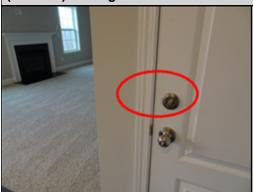
The door lock assembly is not aligned with the striker in the jamb area. The lock could not be engaged to secure the door easily. The door/lock needs repair/replacement to ensure that the door closes securely and operates properly. A general repair specialist or licensed general contractor should be consulted for evaluation and repair.
