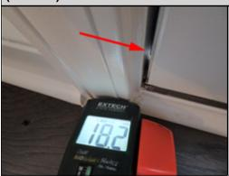
This water stain by the rear door was found to be moist/wet at the time of inspection as measured using a moisture meter tool. Further investigation is needed by a licensed general contractor to determine the extent of the damage. Hidden damage is likely.
