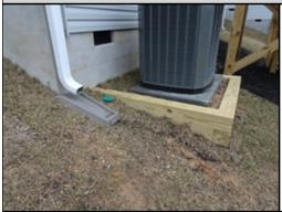
All downspouts should be extended, this one will erode the HVAC retaining wall which will damage the unit.
