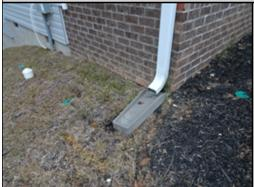
The gutter downspouts are not all effectively extended or piped to direct roof drainage away from the foundation. Direct drainage from the gutter system can result in direct water penetration into the foundation area and foundation deterioration. A licensed general contractor should be consulted for a complete evaluation and to make necessary repairs.
