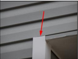
The siding is not flashed on the front left. This should be repaired or replaced by a general contractor to prevent damage from water entry into the wall. Future hidden damage is possible.
