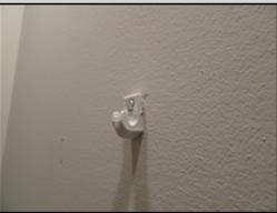
The mirror for the bathroom has been mounted with a fastener that is not typical and is more likely to fail causing the mirror to fall. Broken glass can cause serious injuries. A licensed general contractor should be consulted for a complete evaluation to determine the significance of this concern and make necessary repairs.
