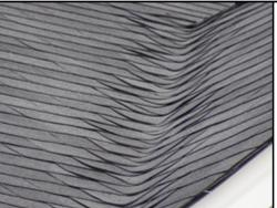
The valleys are woven in a way that runs up the valley more than what is common and is more prone to leak. Also, the singles that do not lay flat are more likely to blow off, tear etc. A roofing contractor should be consulted for a complete evaluation of the roof covering and flashings system to make necessary repairs to ensure the weathertightness of the roof covering system.
