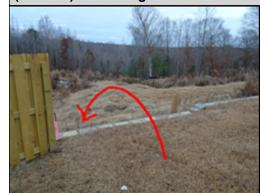
On the back side of the neighboring home, the lot elevation changes. The soil between the levels is retained by a brick retaining wall. There is no guard rail along the wall to prevent a person or animal from falling from the higher front grade to the lower basement level. The absence of a safety railing for a wall of this height presents a safety hazard. A licensed general contractor should be consulted for further evaluation and repair.
