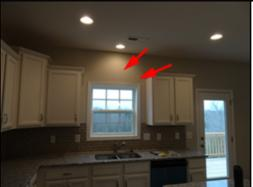
Nail pops were found which mean that the drywall was not properly fastened to the wall. The drywall moves when pressed on. This is not cosmetic. This is incorrect installation of the drywall. This applies to multiple areas of the home. A general repair specialist or licensed general contractor should be consulted for evaluation and repair.
