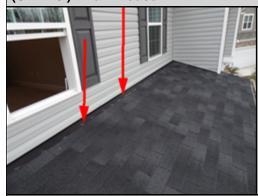
There is no path for ventilation between the lower and upper attic spaces over the front porch. Improper attic ventilation can damage building component such as heat damage to the shingles, void shingle warranty, and result in inadequate conditioning of the living areas when applicable. A licensed general contractor should be consulted for repair/replacement.
