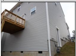
The siding was noted to be installed tightly without leaving room for expansion during summer months. Without proper expansion and contraction clearances the siding may buckle or become loose. A siding installation company or general contractor should be consulted to evaluate and repair the siding to ensure the integrity of the cladding system.
