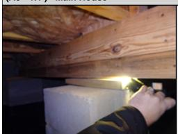
The load of the structure is carried down to the foundation through the floor system. This area under the foyer has a gap which will cause the structure above to sag resulting in drywall pops or more significant concerns. A general repair person or general contractor should be consulted for the repair.
