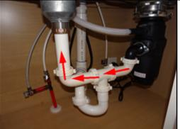
This design shoots water up through the other sink when the disposal runs and then down the drain. A general repair specialist or licensed general contractor should be consulted for evaluation and repair.
