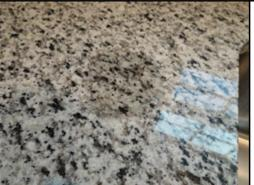
The granite absorbs water which means that the sealing process is not keeping water out of the granite. This means that the granite may become stained if a substance like wine is spilt on the counter top. All of the counter tops in the home should be evaluated and repaired as needed by a general contractor to ensure that all systems are functioning as intended. The contractor should consult specialist in each trade as needed.
